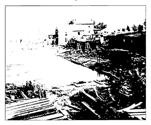
Photo 3 shows the C & O Canal boatyard in Cumberland. On the right, a new boat is being built; in the foreground, processed lumber is stacked in preparation for new construction; and the boats in berths in the background may be for sale or may be in storage after undergoing repairs.
